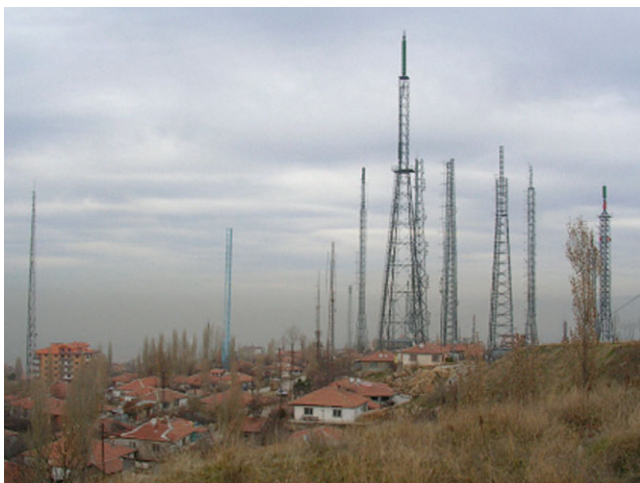
Figure 2 TRT TV transmitter antenna and Private TV, Radio transmitter antennas near the TRT TV transmitter antenna. [Color figure can be viewed in the online issue, which is available at www.interscience.wiley.com ]
